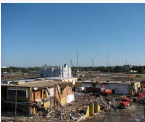
With the last political burdle cleared, demolition and construction moves full speed ahead!
