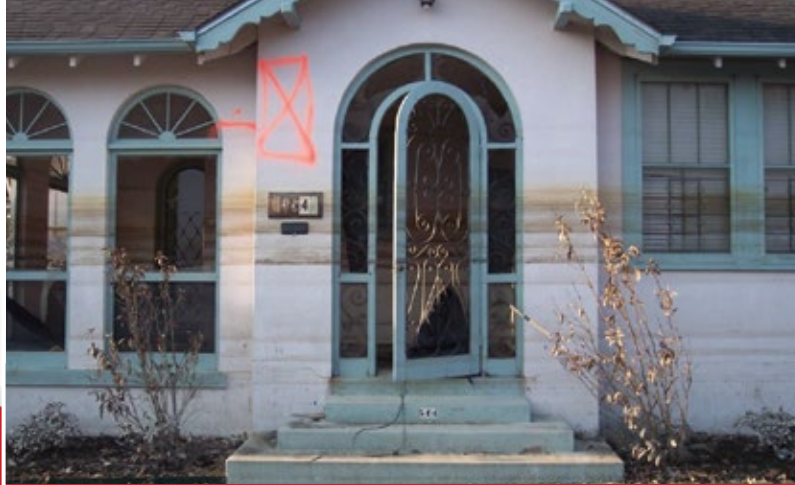
An LSU ENT Resident's home, showing progressive lines of flood waters receding after Katrina. The orange markings were left by National Guardsmen in boats, during their search-and-rescue operations (courtesy Dr. B. Travis).
