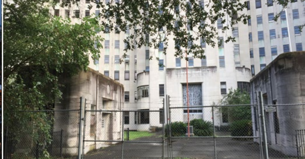
Charity Hospital shuttered and overgrown ten years after Katrina.
